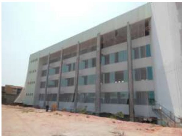
PC-7.1.1 – Fachada frontal (norte)
