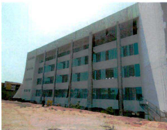
PC-7.1.1 – Fachada frontal (norte)
